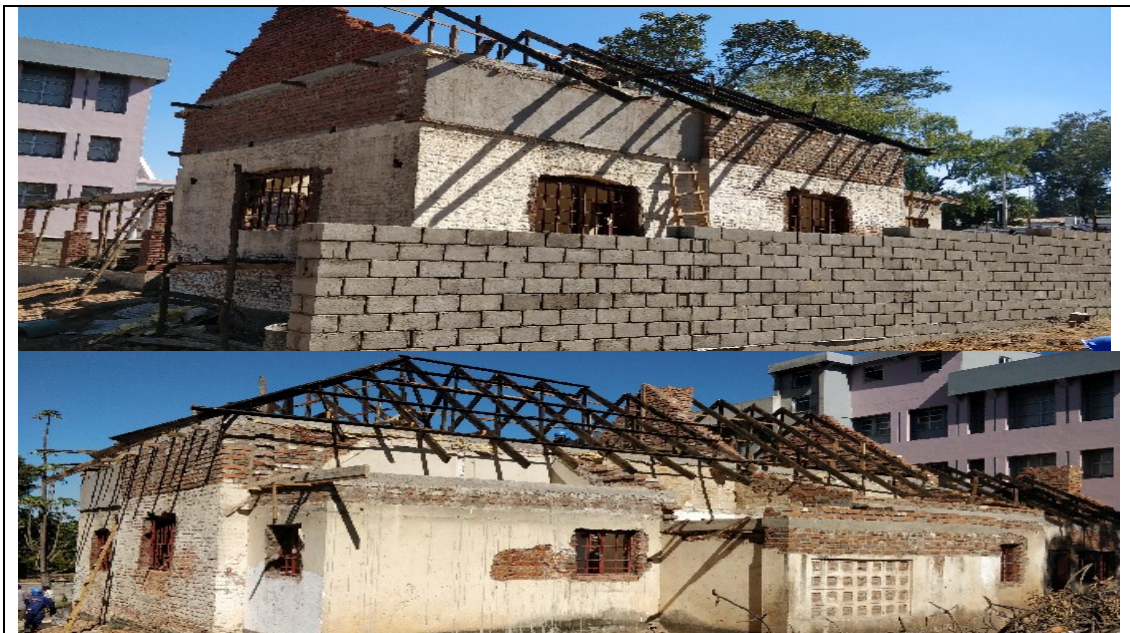
Refurbishment of the Blantyre District Registration Office (DRO) in progress
